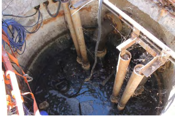
Wet well concrete in fair condition.
