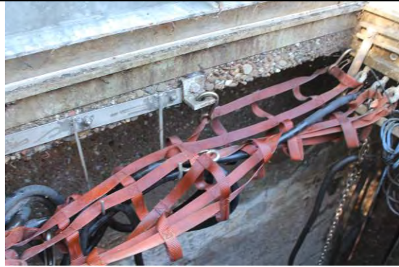
Wet well concrete in poor condition and exhibiting exposed aggregate and H 2 S corrosion.
