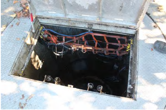
Wet well hatch in fair condition.
