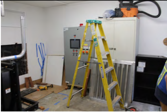
New electrical and I&C being installed during time of the inspection.
