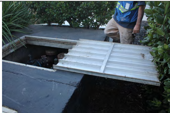
Valve vault in fair condition.
