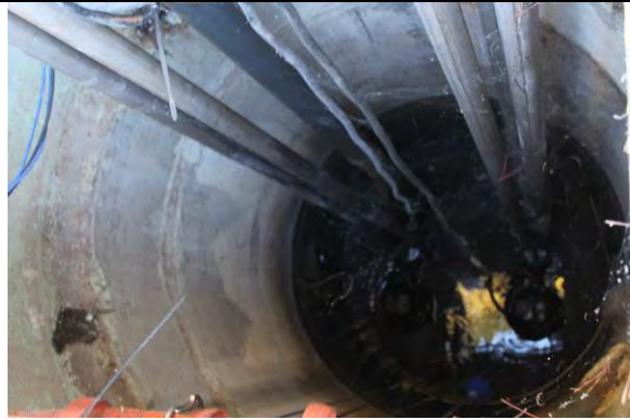
Wet well concrete in fair condition.
