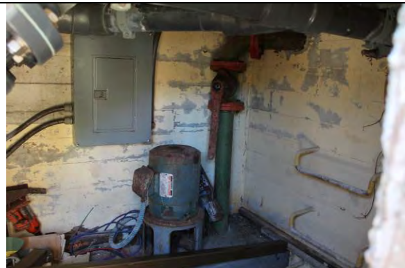
Old lift station.
