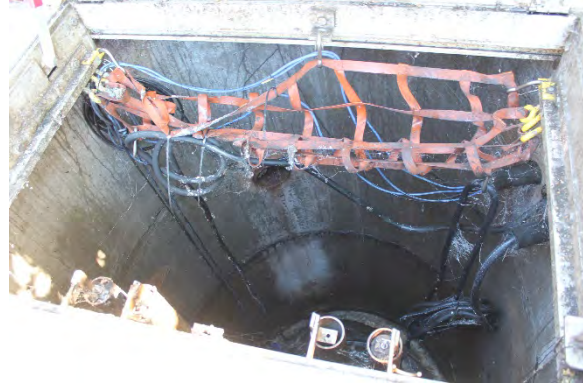
Wet well concrete in good condition.
