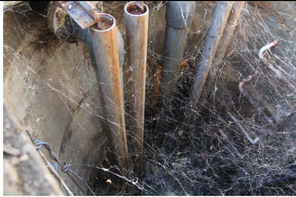
Wet well concrete in fair condition.
