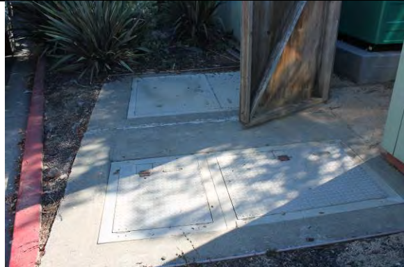
Access hatches to wet well and valve vault.
