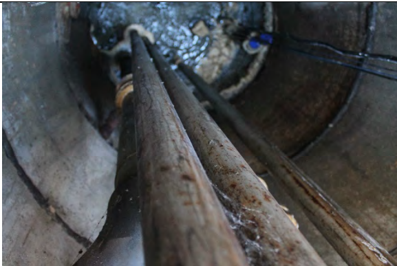
Wet well concrete and submersible pump rails in good condition. Heavy FOG exhibited during inspection.
