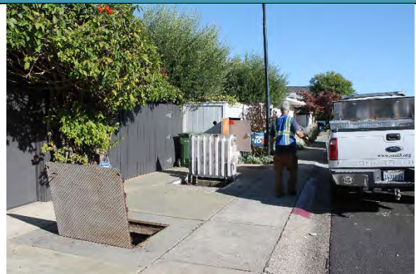
Valve vault (foreground) and wet well (background) access hatches.
