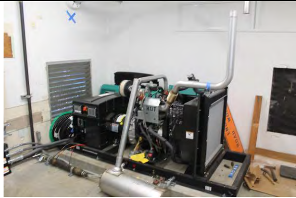
New backup generator being installed during time of the inspection.
