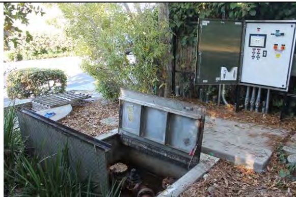
Valve vault concrete and access hatches in fair condition.
