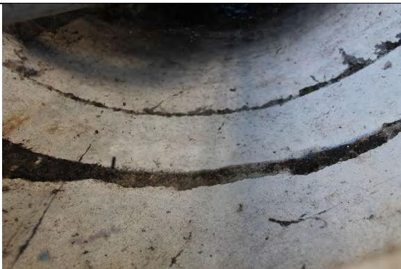
Wet well concrete is in fair condition.
