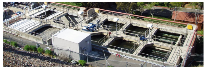
Sanitary District No. 5 of Marin County Main Treatment Facility
