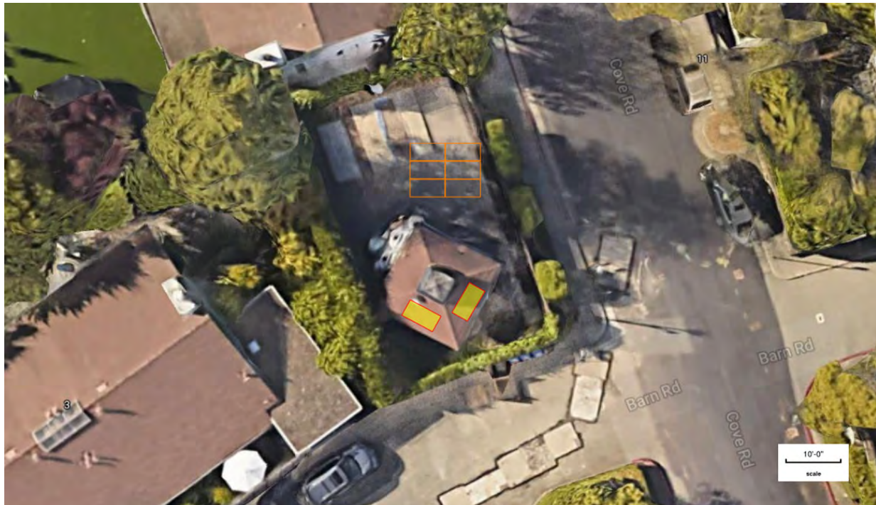
Figure 21 – Belvedere PS-1 PV Potential
