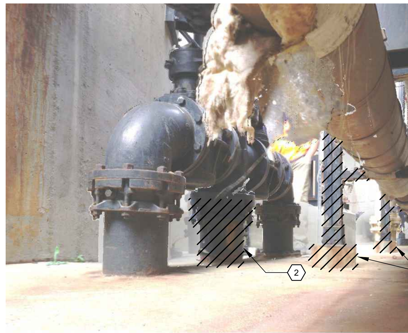
C X101 NTS DEMOLITION PHOTOGRAPH
