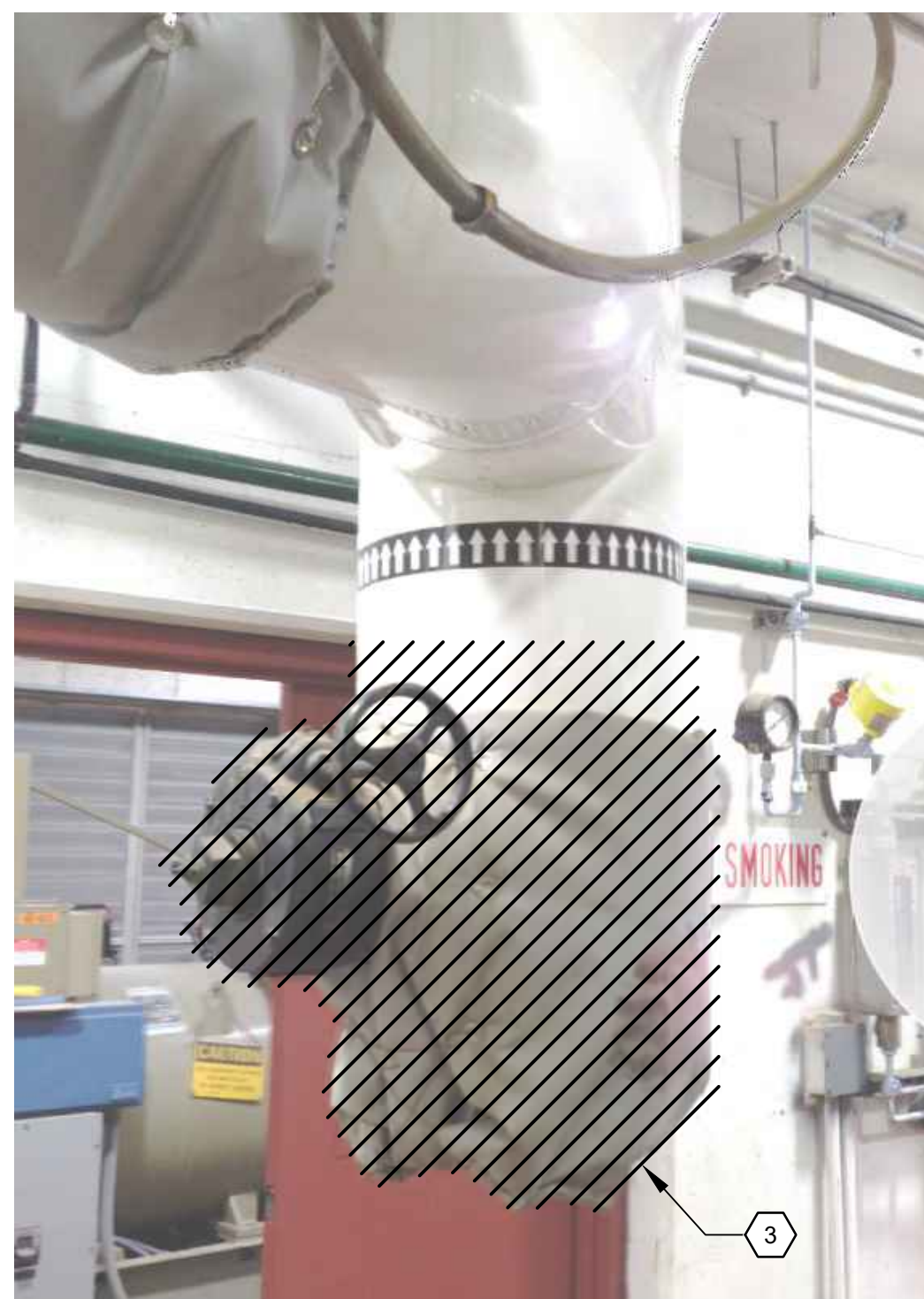
D X101 NTS DEMOLITION PHOTOGRAPH
