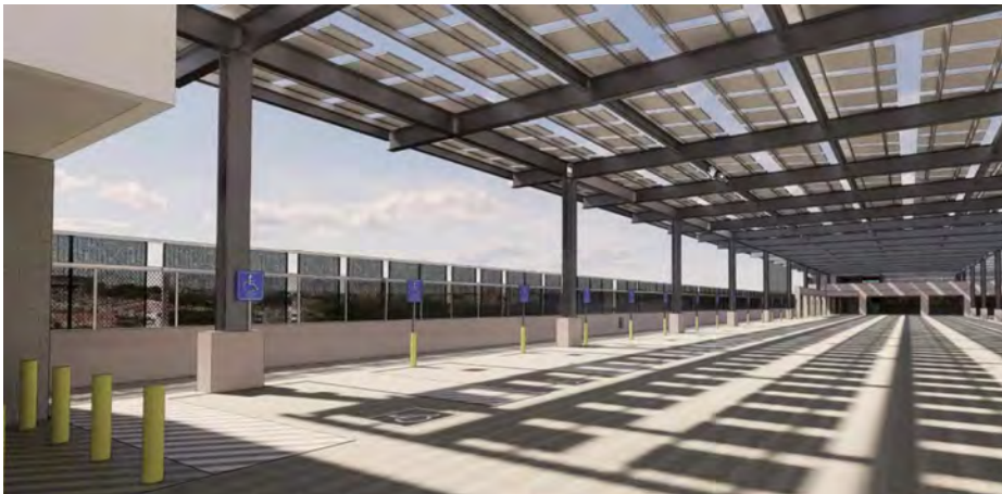
Figure 10 – Example, Canopy Mounted PV System
