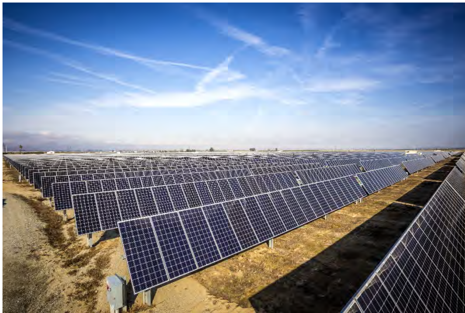
Figure 9 – Example, Ground Mounted PV System
