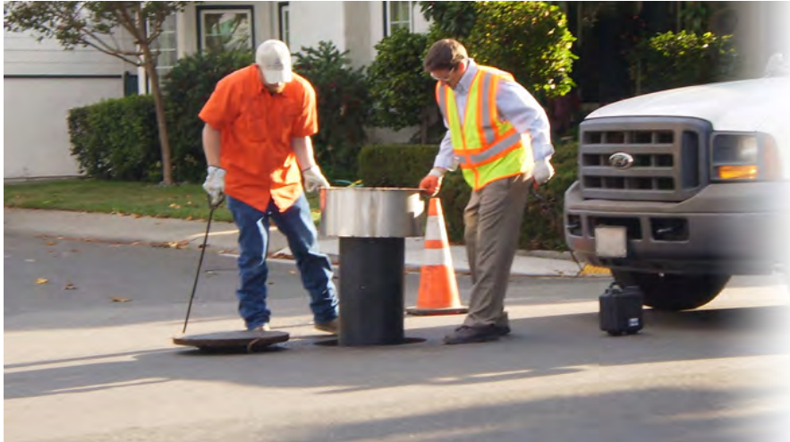
Figure 31. The Mole™ manhole insert with 20 lb. activated carbon to eliminate odors or equivalent device
