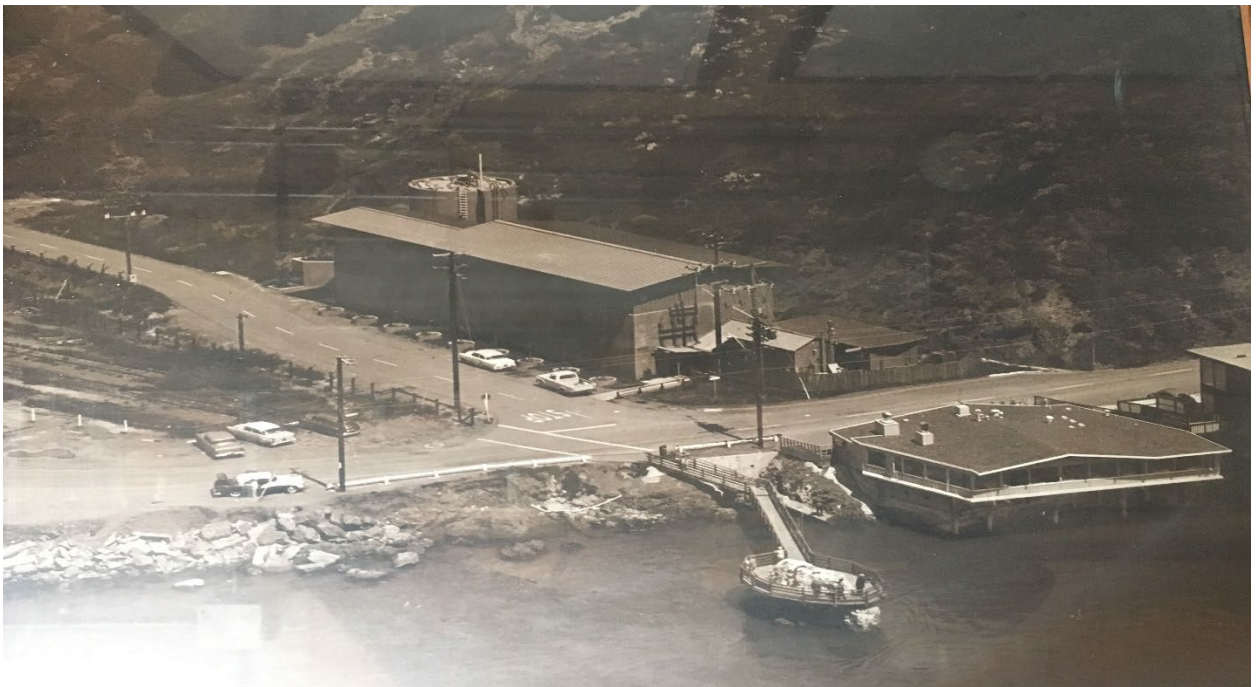
1960's era- Tiburon Peninsula – Wastewater Treatment Plant in service- Primary Treatment only
