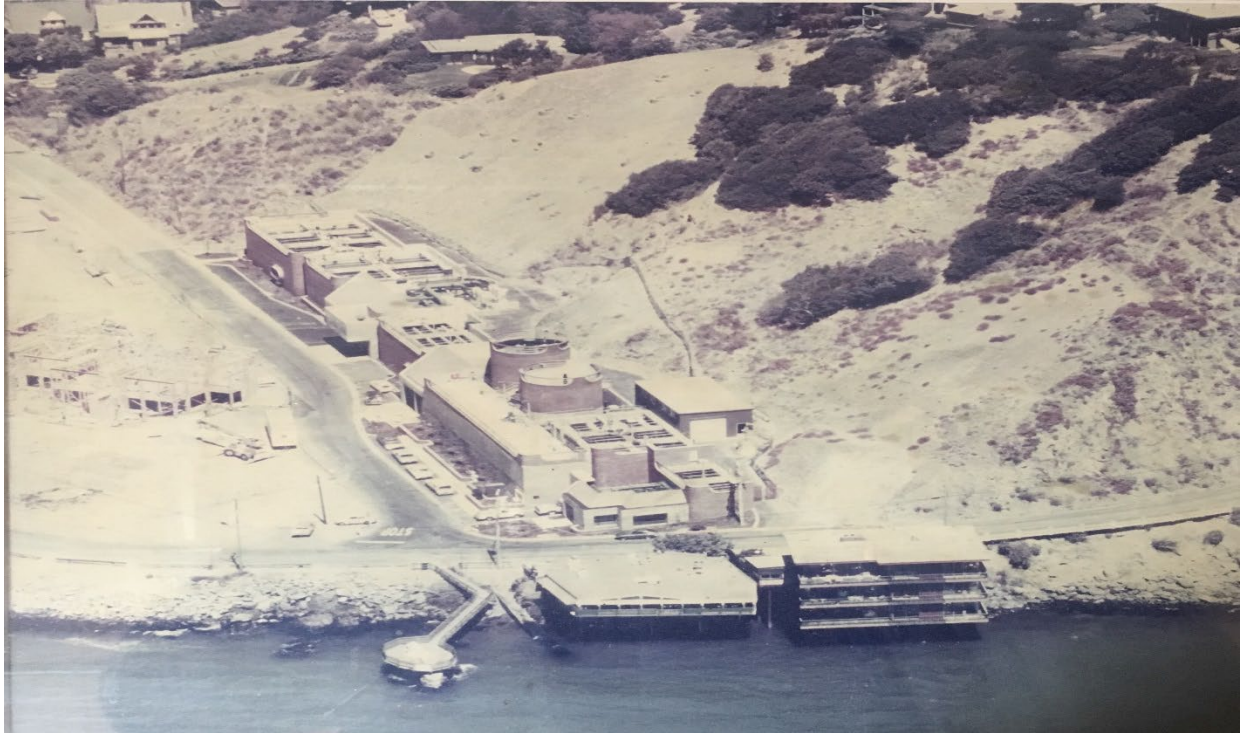
1980's era- Tiburon Peninsula- Secondary Treatment additions to Wastewater Treatment Plant
