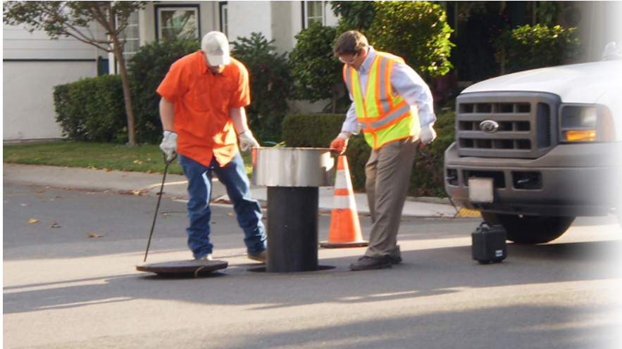
Figure 30. The Mole™ manhole insert with 20 lb. activated carbon to eliminate odors or equivalent device
