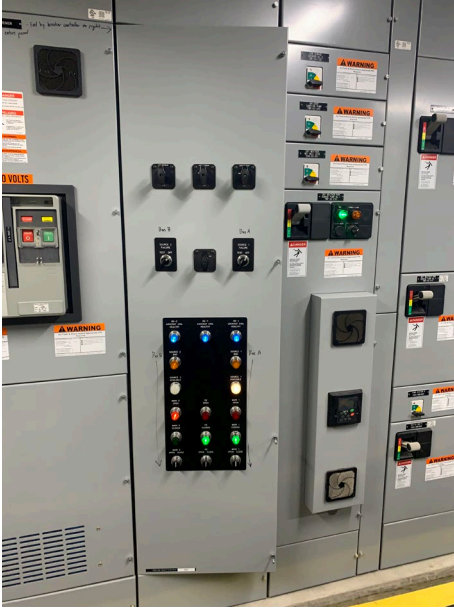
Figure 1: Existing MCC Automatic Transfer Control System Compartment
