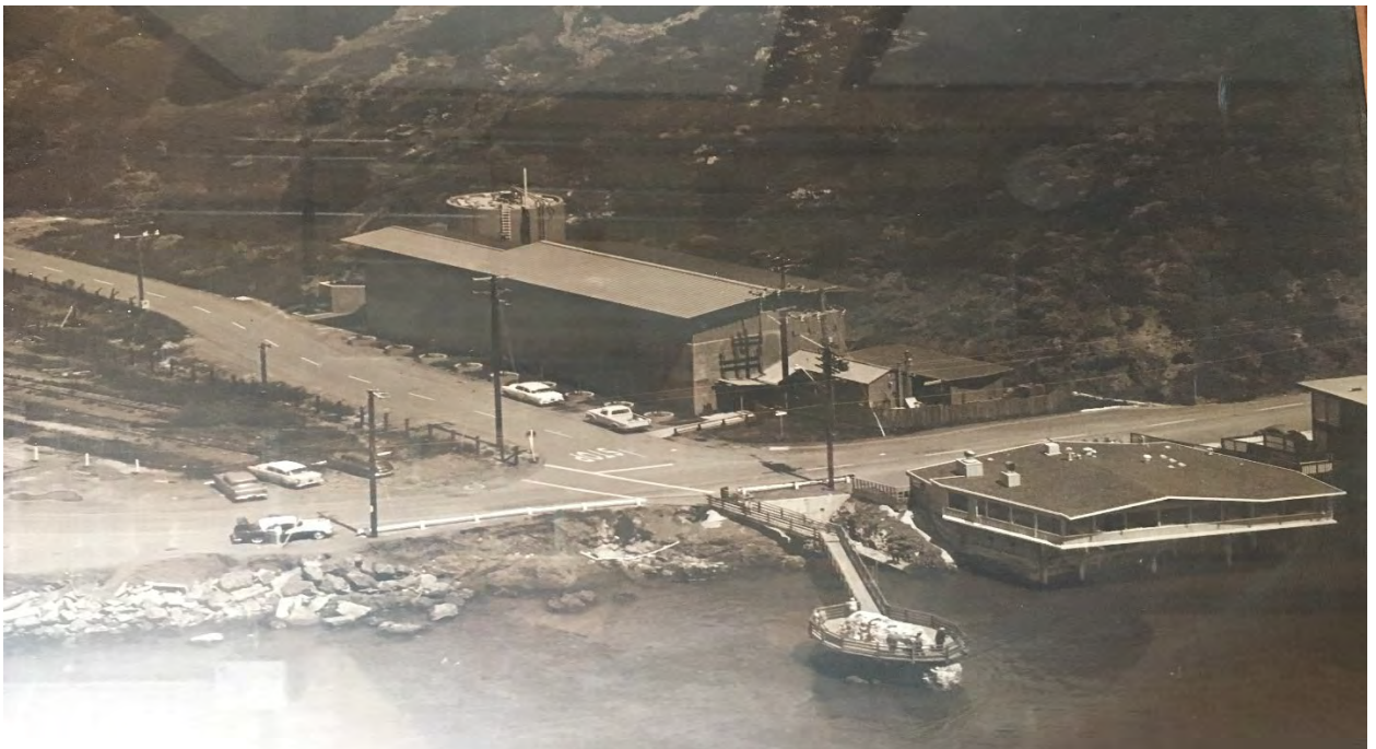
1960's era- Tiburon Peninsula – Wastewater Treatment Plant in service- Primary Treatment only
